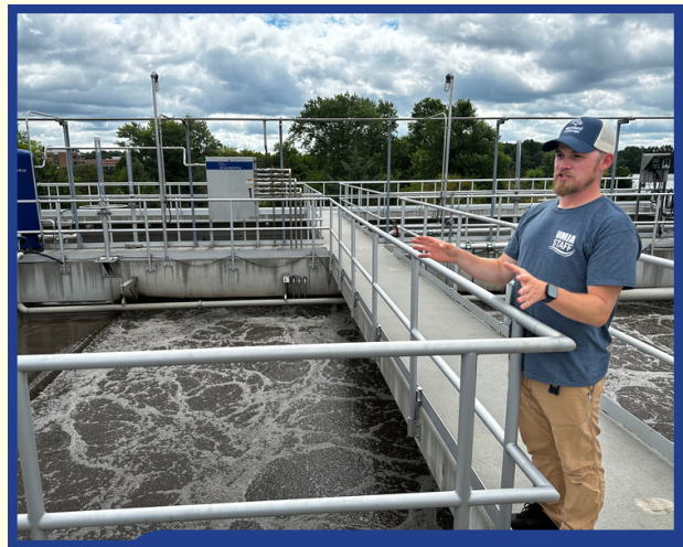
Jason stands above one of several settling tanks where bacteria are at work in treatment water.
