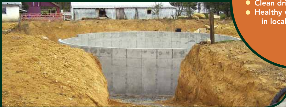
An in-ground liquid manure tank during construction.
