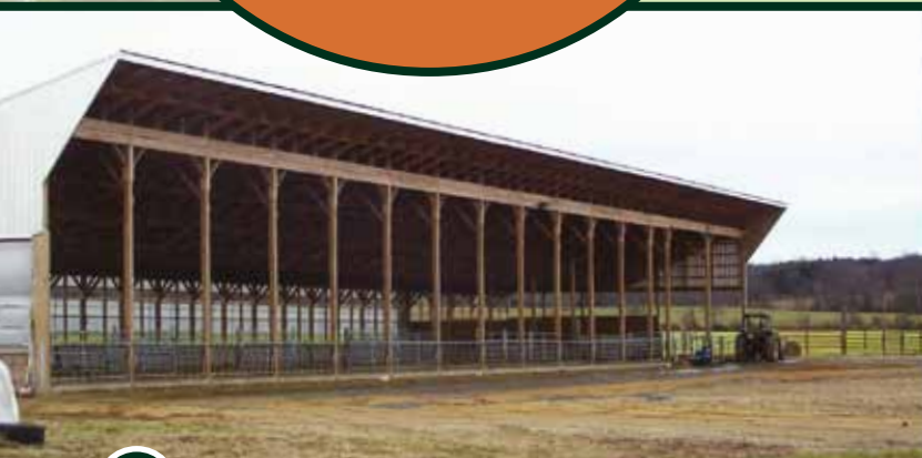
This new structure is designed to store manure for several months.
