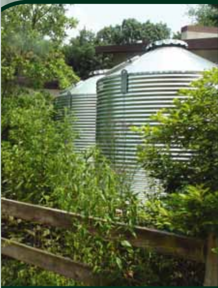
Two cisterns at the Schuylkill Center for Environmental Education in Philadelphia, PA capture runoff from the education building roof.
