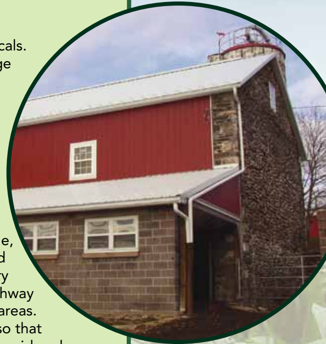
Downspouts should convey water to the downhill corner of the livestock area so the water bypasses areas with waste.
