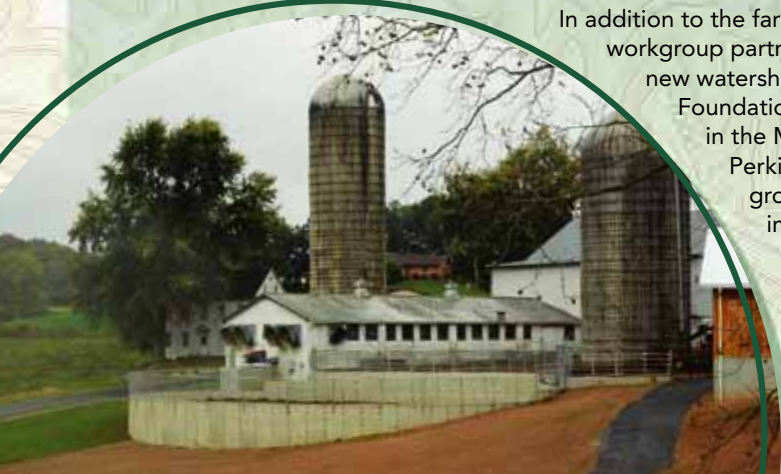
A new manure storage facility was installed at the Davis Farm in Berks County.
